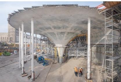
The first of 28 chalice-shaped columns that will combine to hold the roof of Stuttgart's new underground through station was completed in October 2018.
